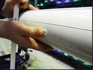
2. Use M6 Hex bolts to secure vertical strips to the beam. Use 1 x plastic washer under the bolt head and 3 x plastic washers between the vertical strip and the beam to act as a spacer.
